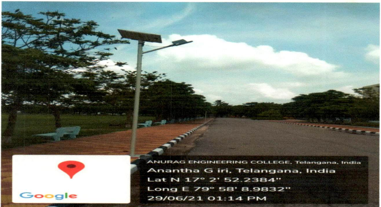
Solar street lights
