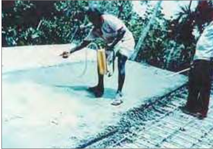
Membrane curing by spraying.
