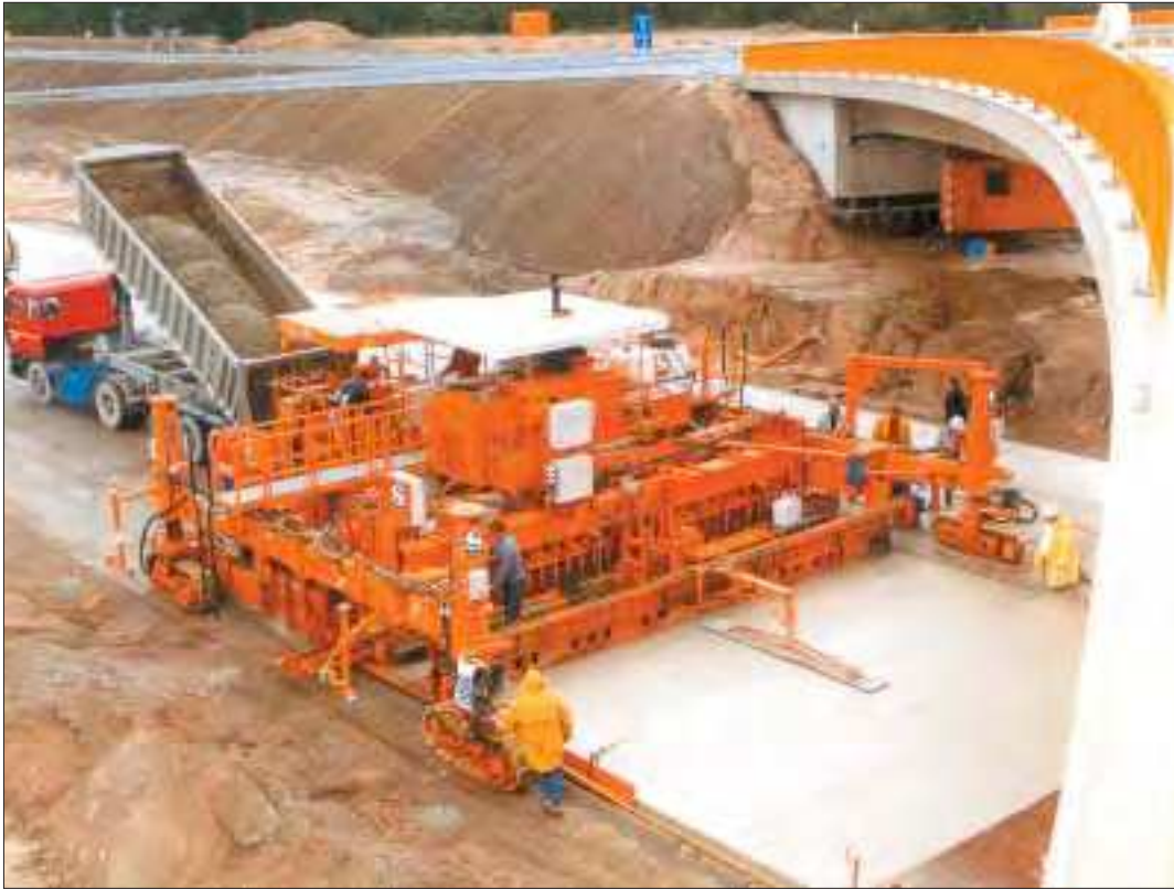
Placing high quality concrete by slip-form technique for a width of 8.5 m.
