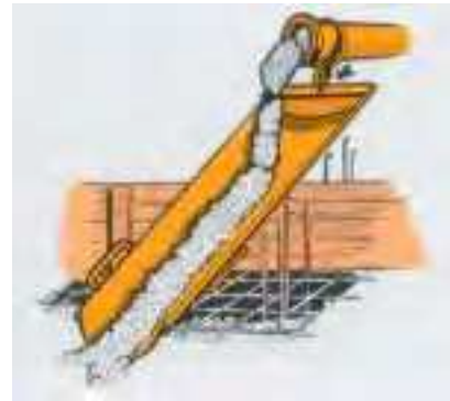
Transporting and placing concrete by chute.
