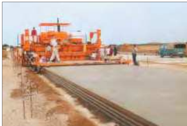
Paving concrete by slip-forming to get sinusoidal profile for linking with the adjacent slab.
