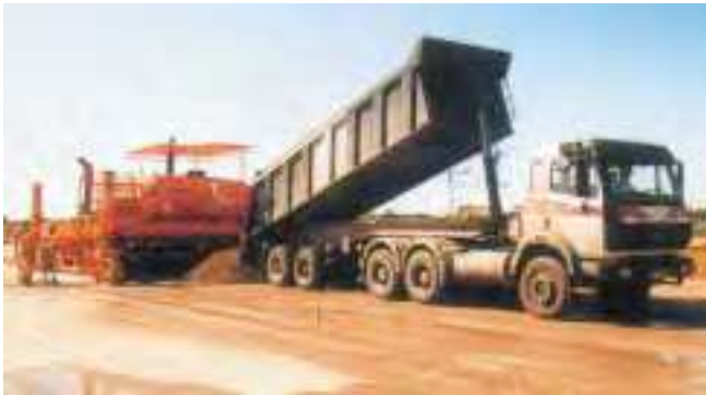
Truck mixer and dumper for transporting stiff concrete
