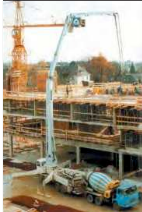
Placing concrete by pump and placing boom.
