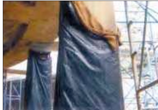
Curing vertical surface by wet covering.
