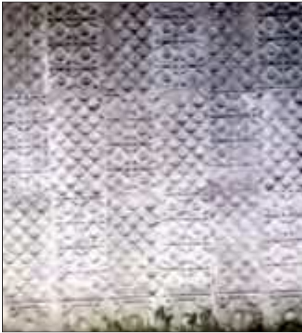
Applied finish work done at CME
