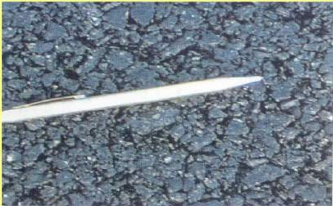
Freshly Laid BC layer
