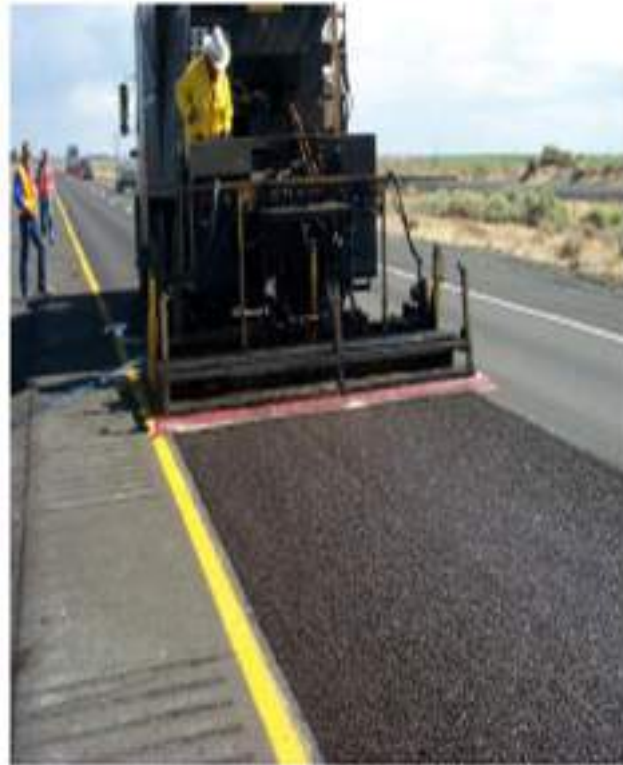
Figure 2. Microsurfacing placement.
