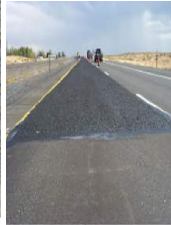
Figure 4. Finished microsurface.
