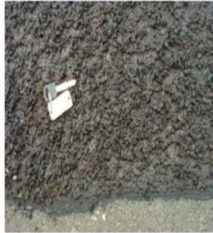
Figure 3. Microsurface close-up.
