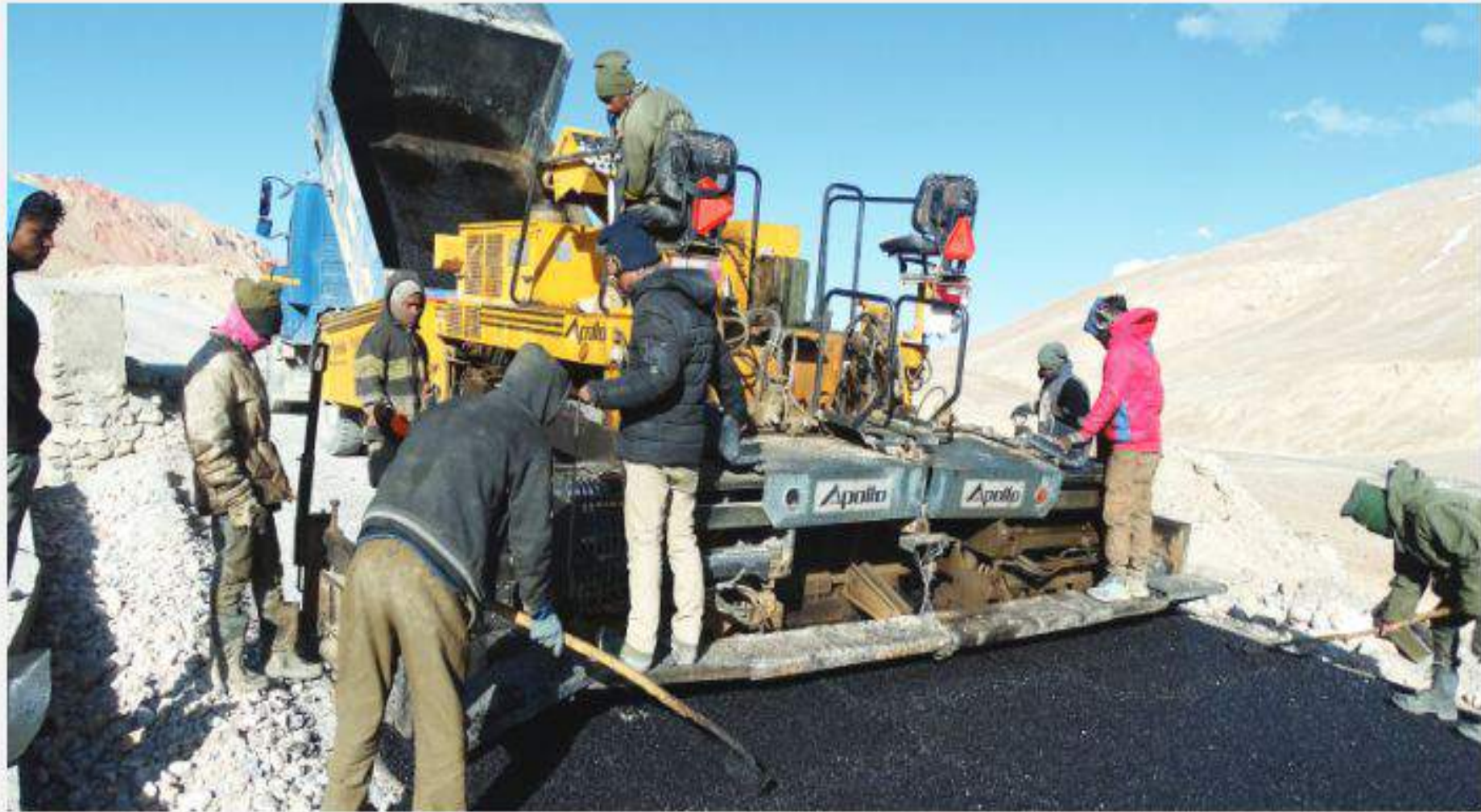
Man and machine working in tandem to blacktop the world's highest motorable road in Eastern Ladakh at 19,024 ft.
