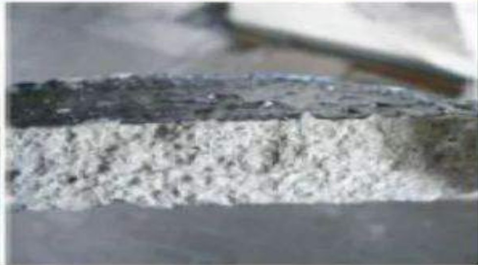
Good Surface, Poor Penetration
