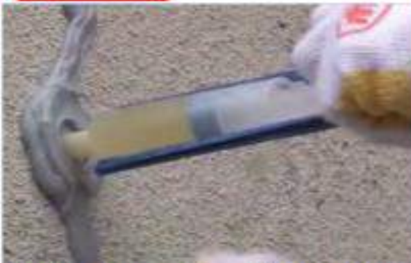
Injection into cracks with epoxy resin
